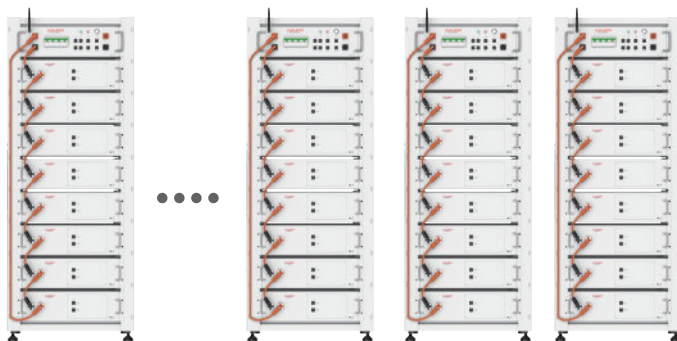
Expansion in DC side
